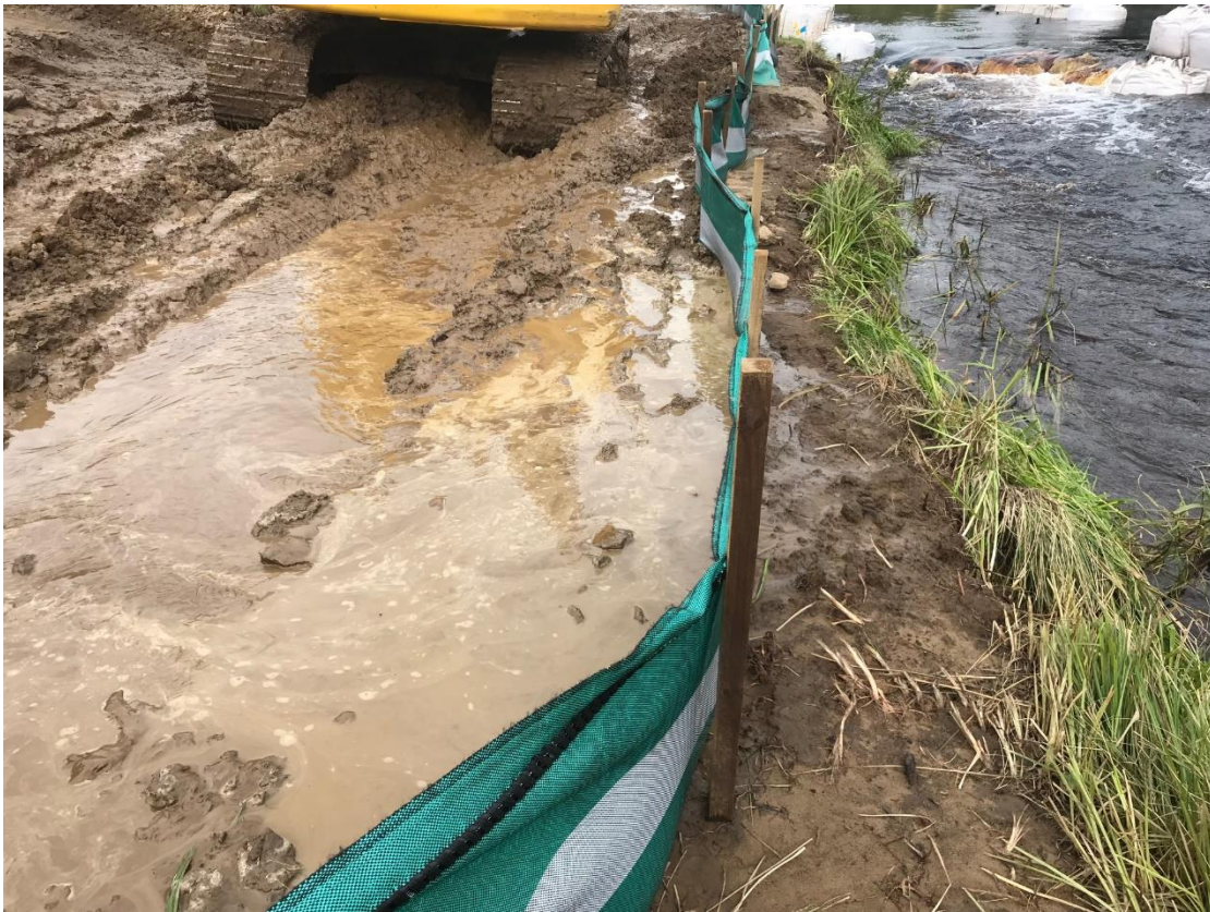
Figure 5.8 Terrastop silt fence installed on a riverbank preventing silt and soiled water reaching watercourse
