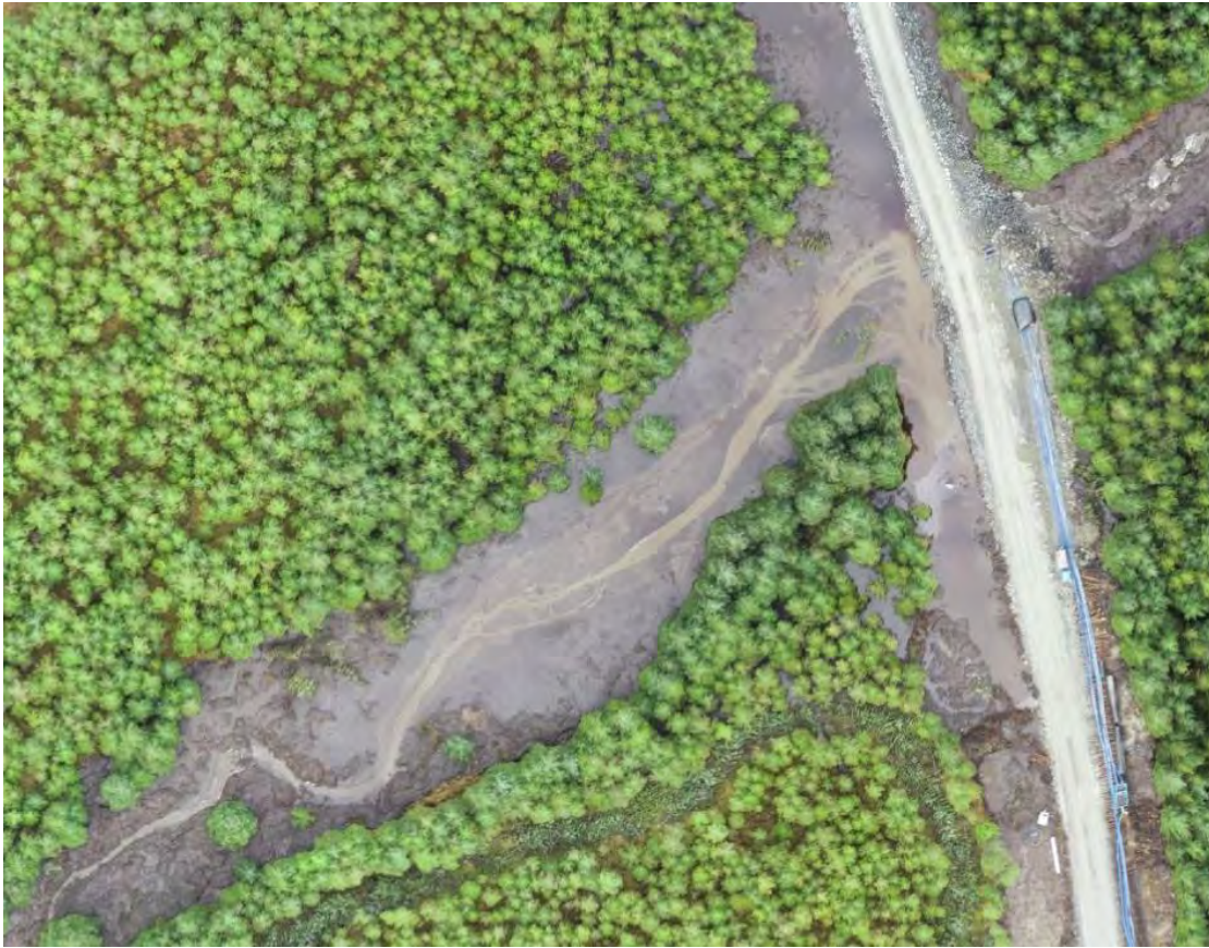
Figure 2.2 Aerial image of water and peat impoundment area upstream of Wall 1 showing large volumes of impounded peat and clearly identifiable channel for water reaching Wall 1
