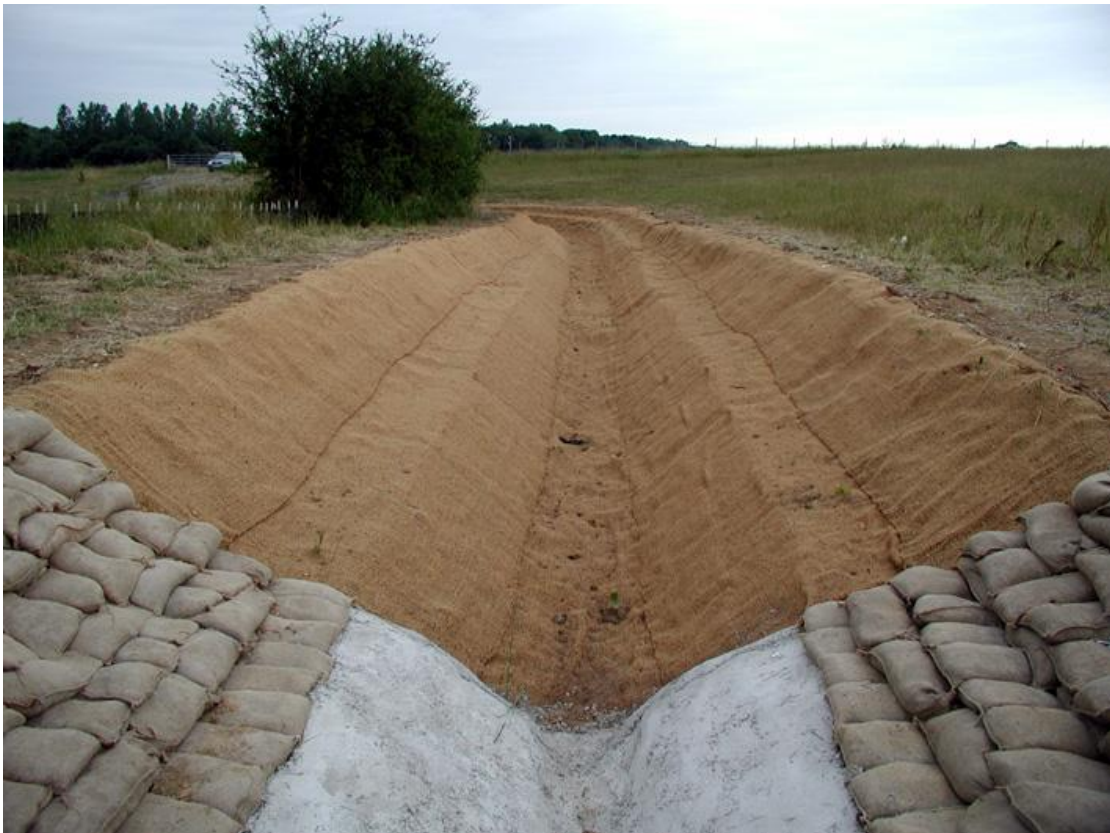
Plate 5.17 Large-scale use of CoriMesh to establish vegetated surfaces on drainage channel embankments
