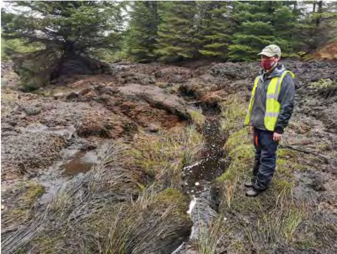
Figure 5.13 Area of heavier peat deposits in Reach 4 (facing upstream) where temporary silt fencing is recommended. Immediate streamside zone is largely free of peat.
