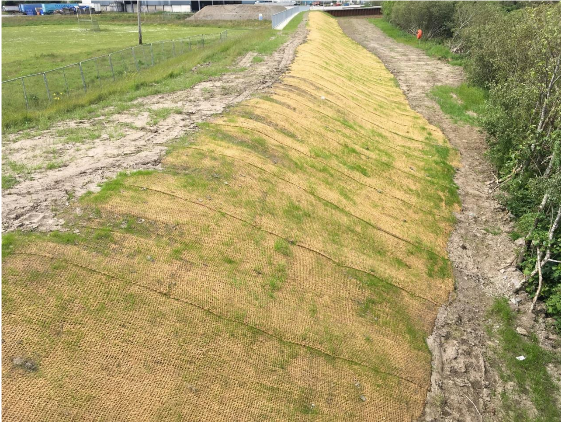
Plate 5.16 Large-scale use of CoriMesh to stabilise exposed ground, as likely required upstream of Wall 1 once large peat deposits are removed
