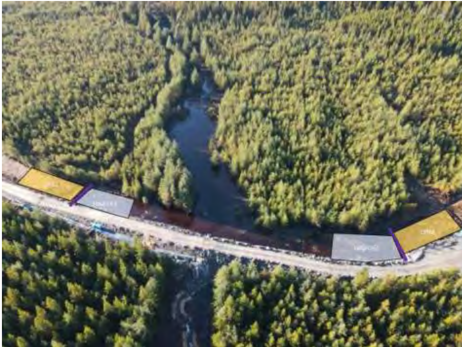
Figure 5.14 Creation of outer drying cells
