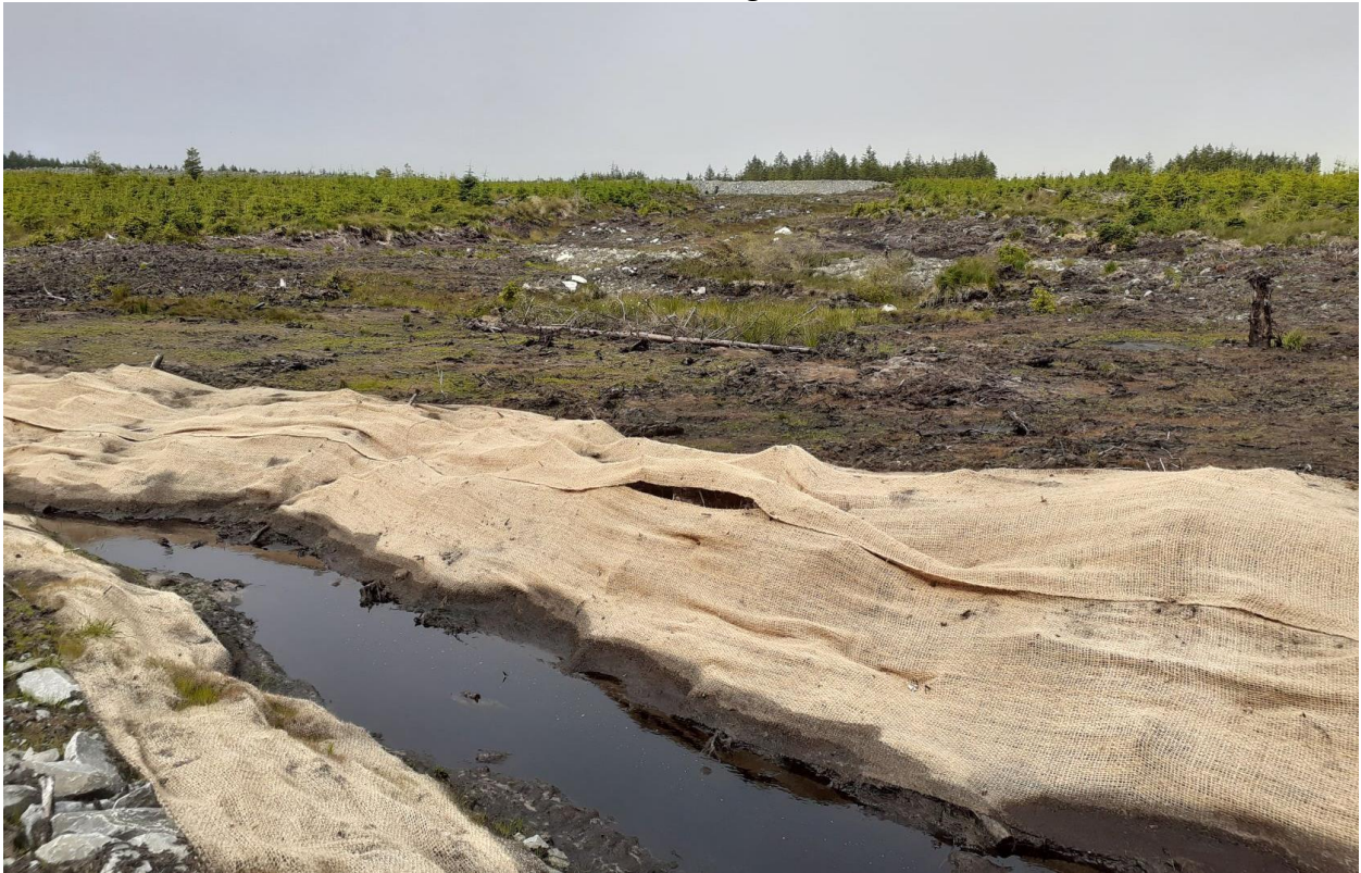
Photo 5 - Sruhingarve stream, looking up towards Wall 3, 8/7/22
