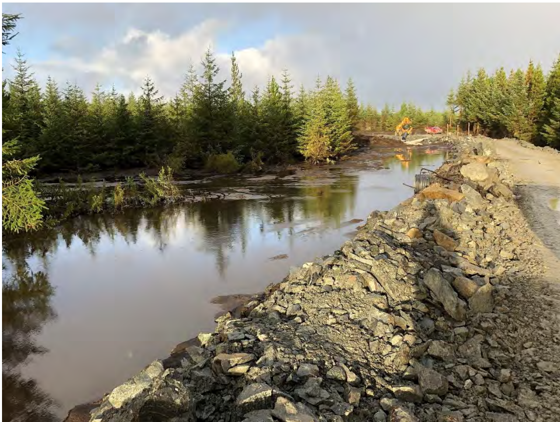
Figure 2.1 Water and sediment impoundment area upstream of Wall 1 showing stabilised situation and deposits of peat up to surface of water
