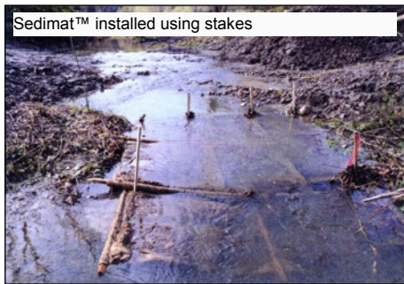
Disturbed sediment entering Sedimat™
