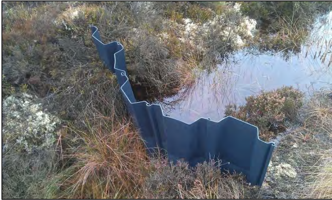
Plate 3.1 Example of plastic dams to be used for on-site drain blocking.
