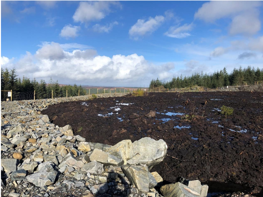
Plate 2.2 Completed peat cell at borrow pit southwest of T12
