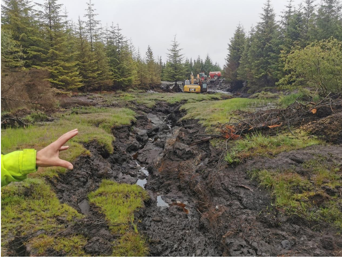
Plate 2.4 View of impounded area during sediment removal works, facing downstream
