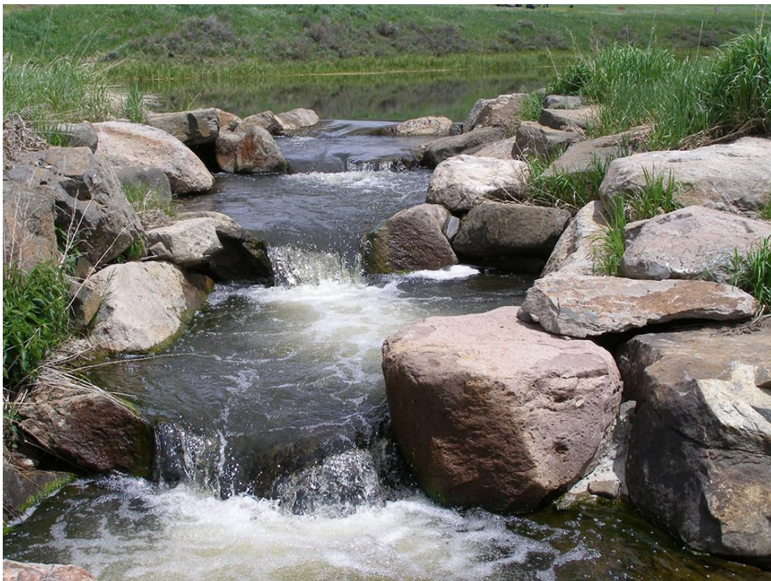
Plate 3.1 Example of Rock Step Pool Structure
