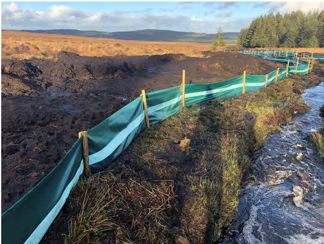
Figure 5.10 Silt fence Installed on Reach 4
